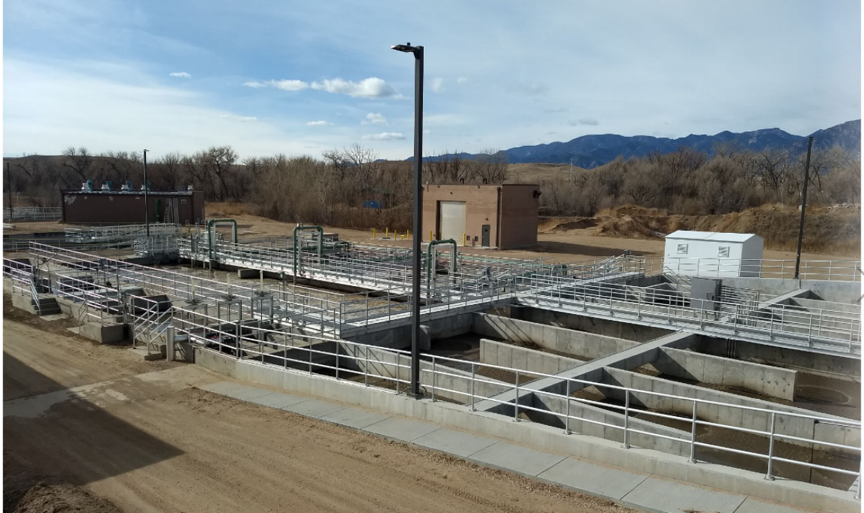
Aerial view of bio nutrient removal basins.
