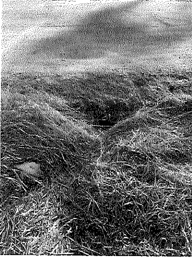
Figure 41: Upstream end Culvert 3
