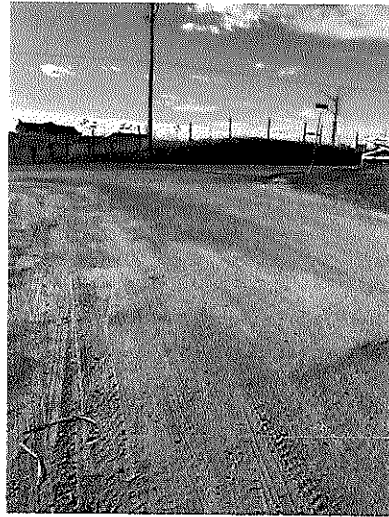
Figure 45: Herring Road Intersection
