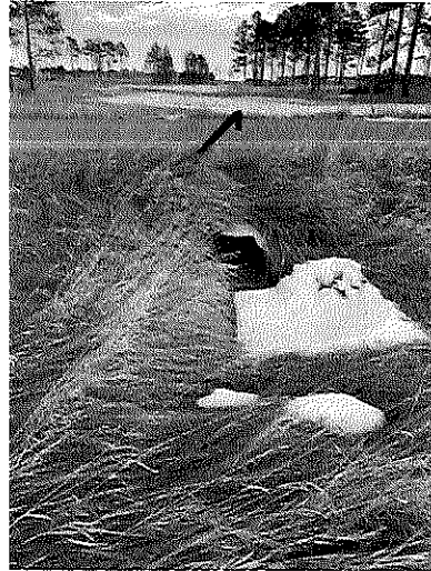
Figure 55: culvert under Herring
