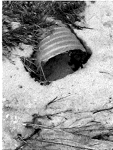
Figure 56: Culvert under Herring
