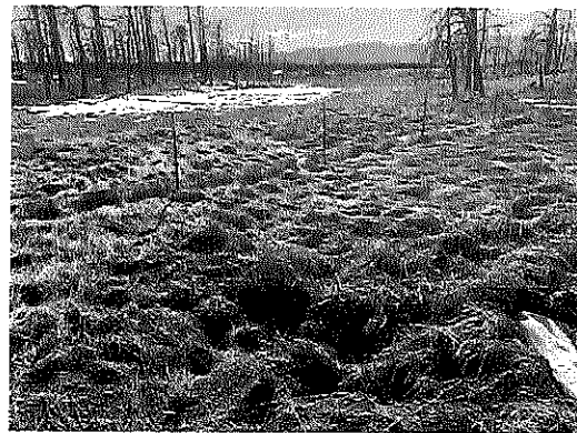
Figure 6: Facing downstream of Culvert 1
