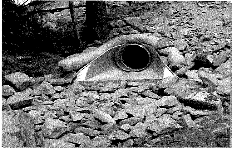
Photograph TOP-1. Riprap outlet protection.
