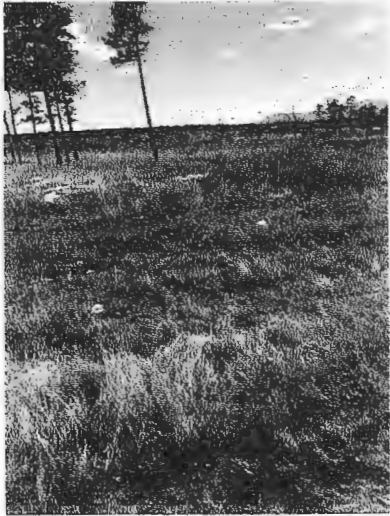
Figure 52: Facing downstream of culvert 2
