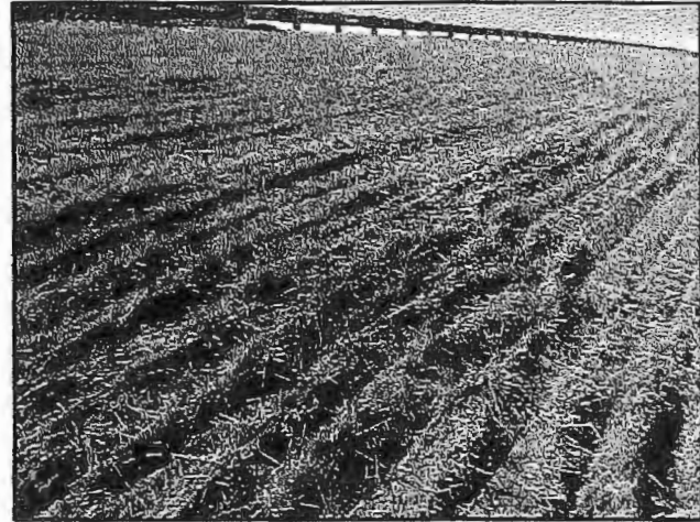
Straw Mulching on disturbed side slope
