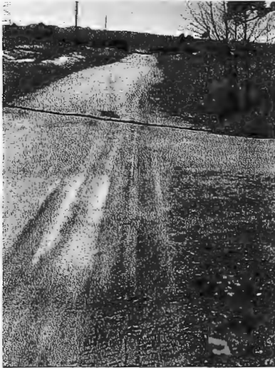
Figure 8: Facing west along northerly edge of road
