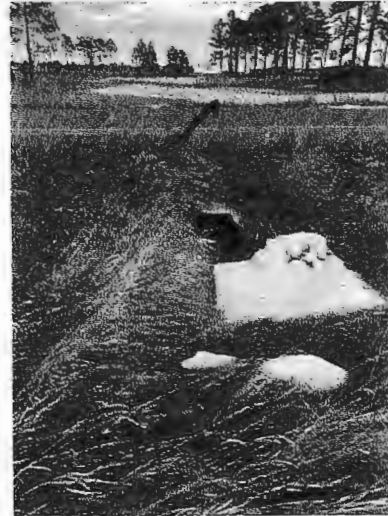
Figure 55: culvert under Herring
