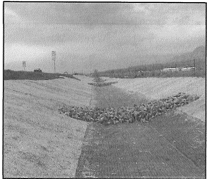
Rock check dam along lined drainage ditch
