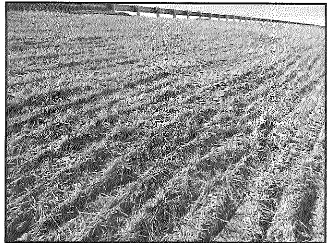
Straw Mulching on disturbed side slope
