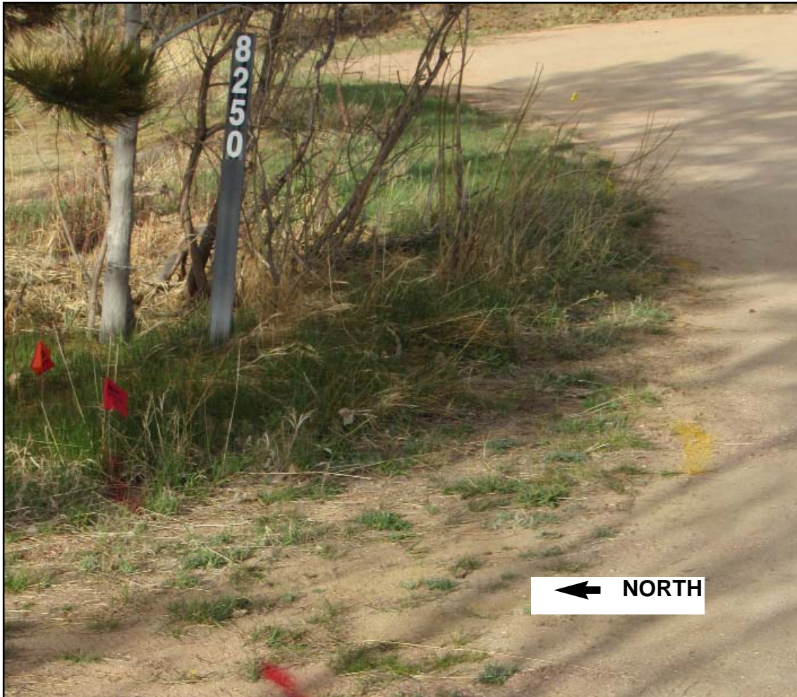
NE edge of 8250 drive at intersection with FHC. Note the red flags for phone-service and also the yellow paint and westernmost of the two yellow flags on the north side for gas.
