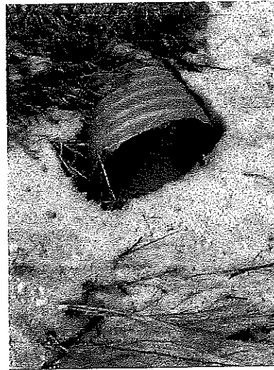
Figure 56: Culvert under Herring
