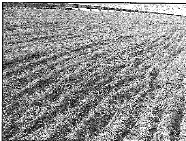
Straw Mulching on disturbed side slope
