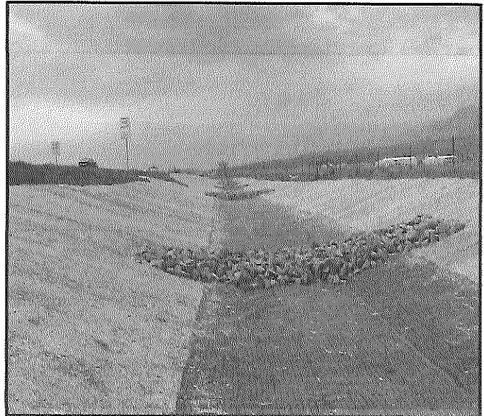
Rock check dam along lined drainage ditch
