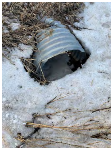
Figure 56: Culvert under Herring
