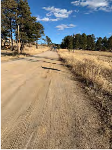
Figure 46: Facing east of intersection
