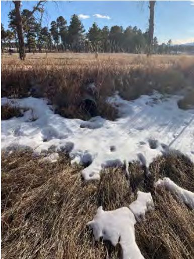
Figure 48: 18" CMP under Drive
