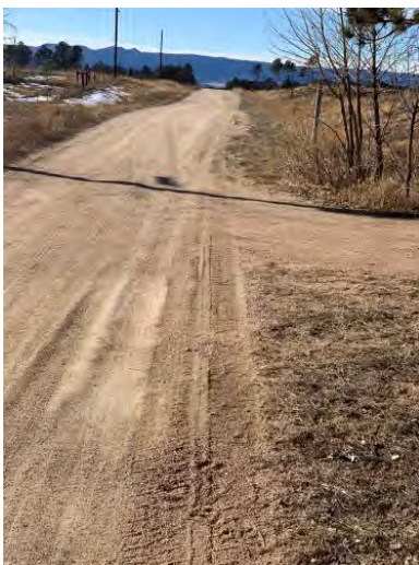
Figure 8: Facing west along northerly edge of road
