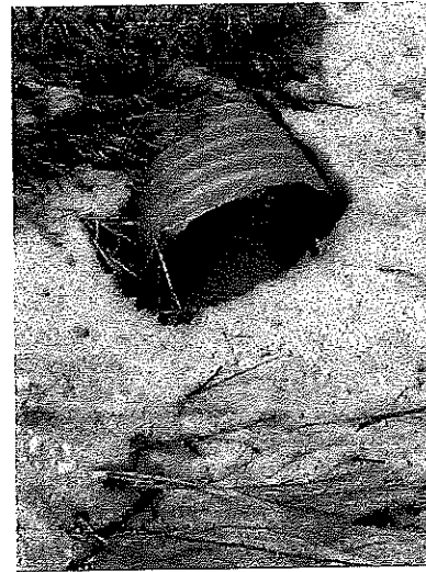
Figure 56: Culvert under Herring
