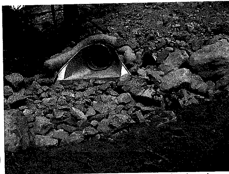
EROSION LOG CULVERT OUTLET PROTECTION
