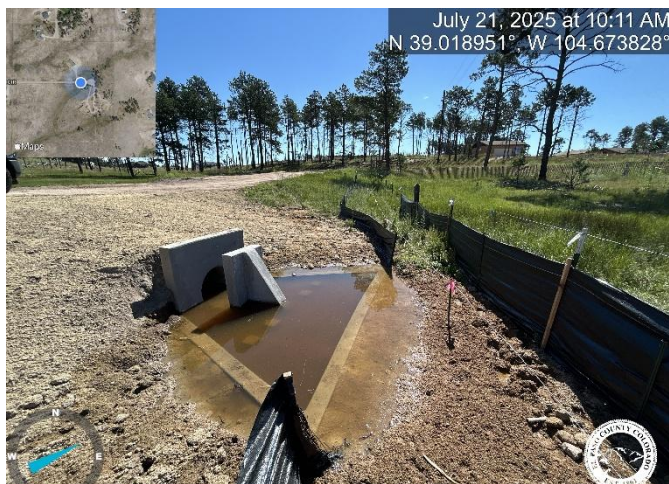
Photo 2: Ensure positive drainage from new headwall.
