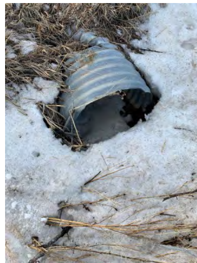
Figure 56: Culvert under Herring
