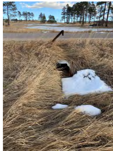
Figure 55: culvert under Herring
