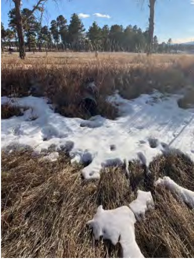
Figure 48: 18" CMP under Drive
