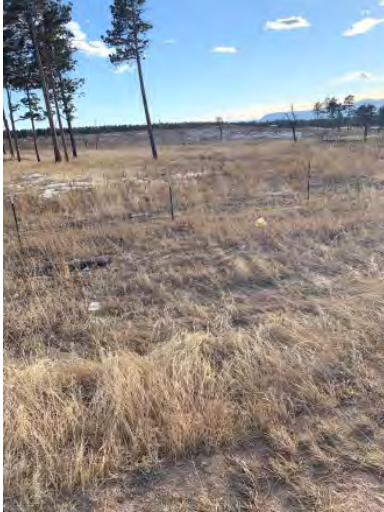
Figure 52: Facing downstream of culvert 2
