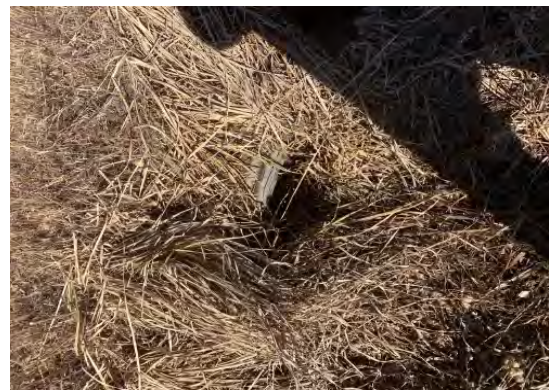
Figure 5: Downstream End of Culvert 1
