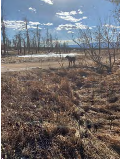
Figure 1: Upstream End of Culvert #1
