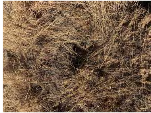
Figure 43:Downstream end of Culvert 3
