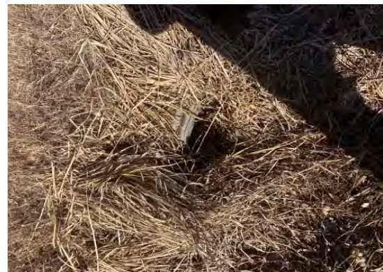
Figure 5: Downstream End of Culvert 1
