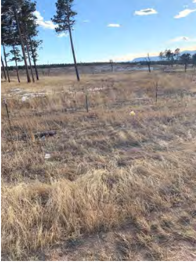
Figure 52: Facing downstream of culvert 2
