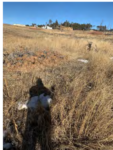
Figure 22: Facing NE of Culvert 2
