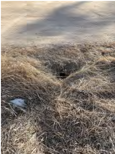
Figure 41: Upstream end Culvert 3
