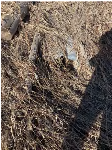
Figure 24: Downstream end of Culvert 2
