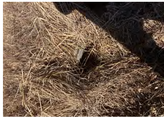
Figure 5: Downstream End of Culvert 1
