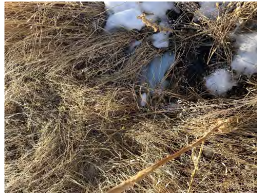
Figure 21: Upstream end of Culvert 2
