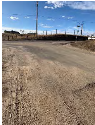
Figure 45: Herring Road Intersection
