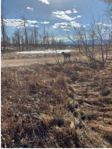
Figure 1: Upstream End of Culvert #1
