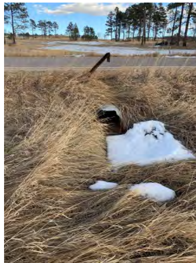
Figure 55: culvert under Herring
