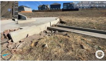
Photo 3: Pond C5: Remove sediment and debris from outlet structure micropool.
