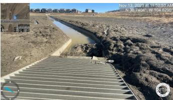
Photo 1: Pond C5: Raise pond bottom to top of trickle channel curb with a 3% slope towards trickle channel for positive drainage.
