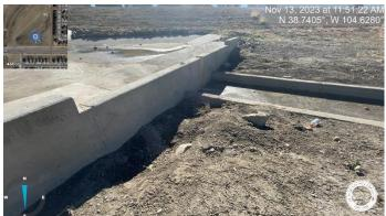
Photo 5: Pond C5: Fill in undercut areas on Forebay A and B.
