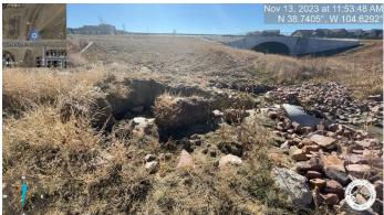
Photo 9: Pond C5: Repair blowout about outlet pipe and implement stabilization.
