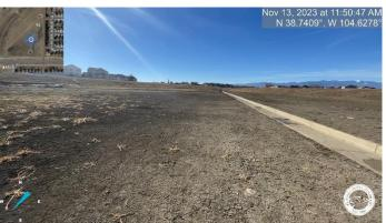
Photo 7: Pond C5: Failure to achieve uniform vegetative cover with an individual plant density of at least 70 percent in pond bottom.
