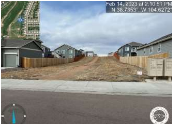
Photo 13: Remove temporary control measure (straw wattle) from all Tract areas.
