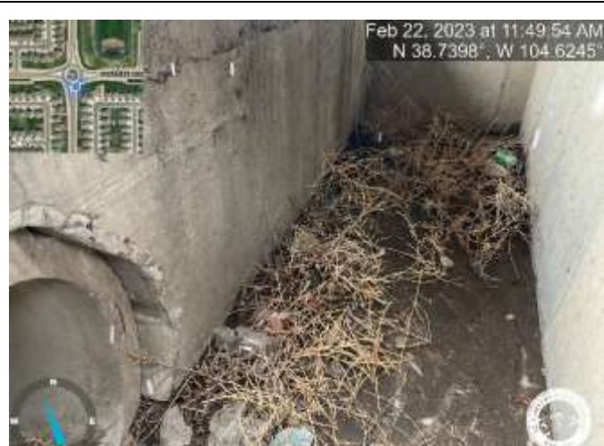
Photo 18: Inlet DP-30: Remove sediment and debris from inlet (inlet is marked with a green dot on the lid).
