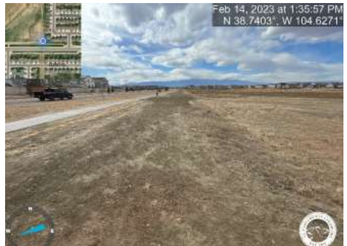
Photo 8: South perimeter of Pond C5: Failure to achieve uniform vegetative cover with an individual plant density of at least 70 percent.
