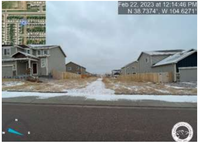
Photo 14: Remove temporary control measure (straw wattle) from all Tract areas.
