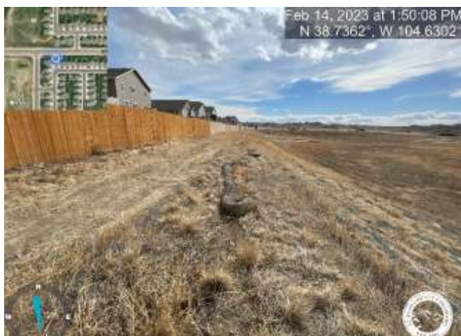
Photo 12: Remove temporary controls measures along the east perimeter.
