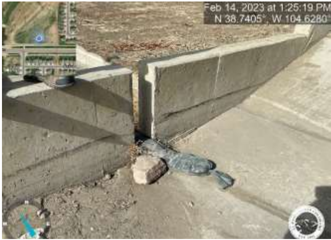
Photo 5: Pond C5: Remove rock sock from forebay notch.
