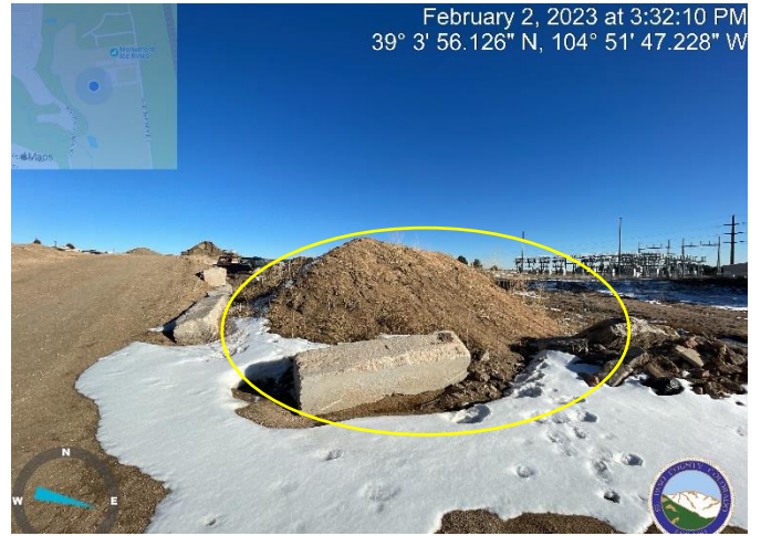
Photo 6: Remove stockpiles south of maintenance access road.
