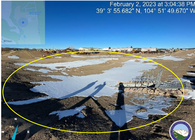
Photo 1: Stabilize entire Pond.
