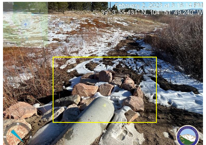
Photo 4: Install riprap pad at outlet pipe per plan.
