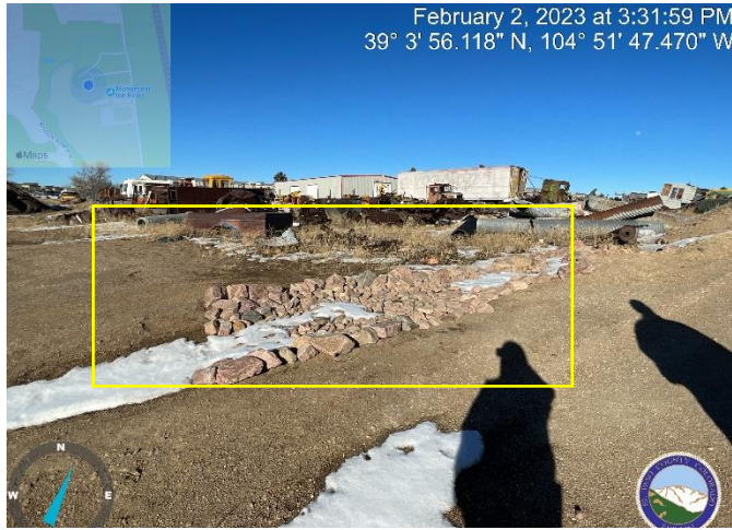
Photo 5: Verify riprap rundown in As-Built Drawings.
