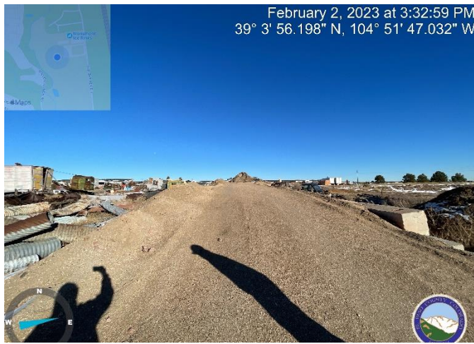
Photo 7: Verify length and slope of maintenance access road in As-Built Drawings.
