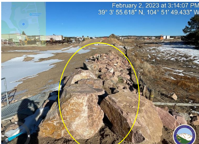
Photo 3: Install emergency spillway riprap per plan.
