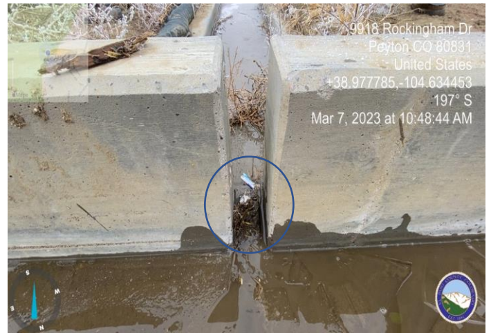
Photo 6: Remove excess concrete from forebay weir notch which is restricting flow.
