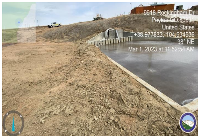
Photo 3: Remove sediment near forebay and grade pond bottom to slope 3% towards the forebay to promote positive drainage.
