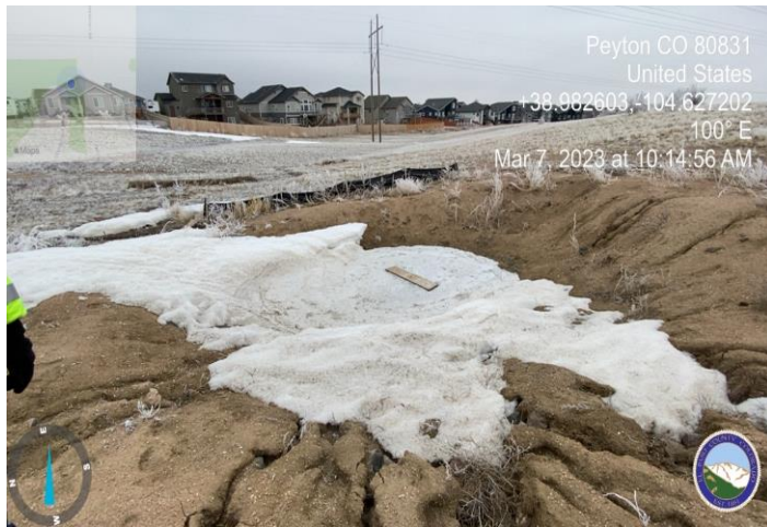
Photo 5: Waterloo cul-de-sac requires 9" riprap. Regrade and install per plan detail
