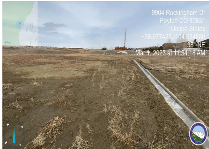
Photo 1: Lower pond bottom to top of trickle channel curb with a 3% slope towards trickle channel to promote positive drainage.
